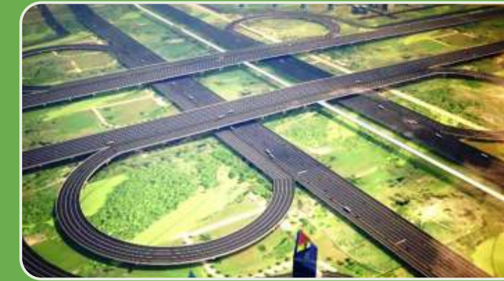
250 M WIDE 6 LANE AHMEDABAD-DHOLERA EXPRESS WAY
